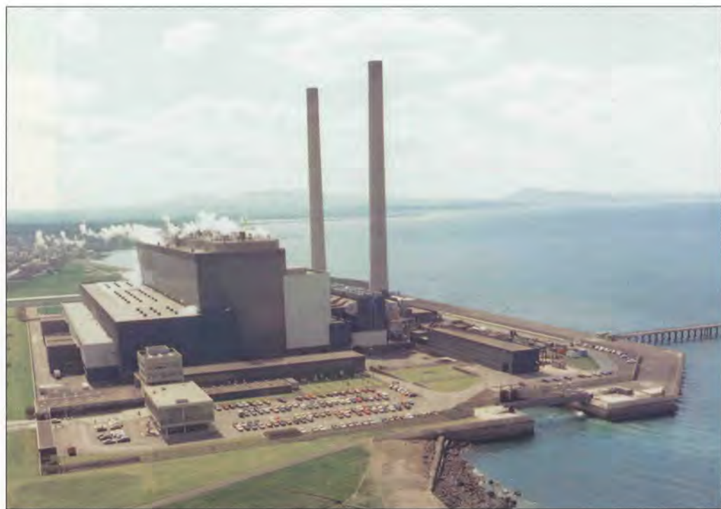
Longannet Power Station.
