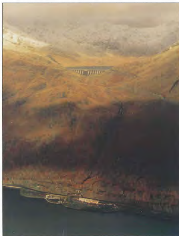
Cruachan Power Station.
