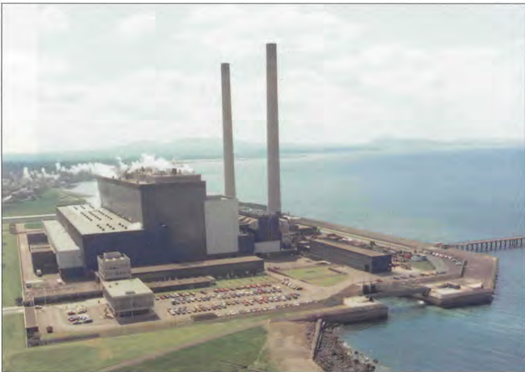
Longannet Power Station.
